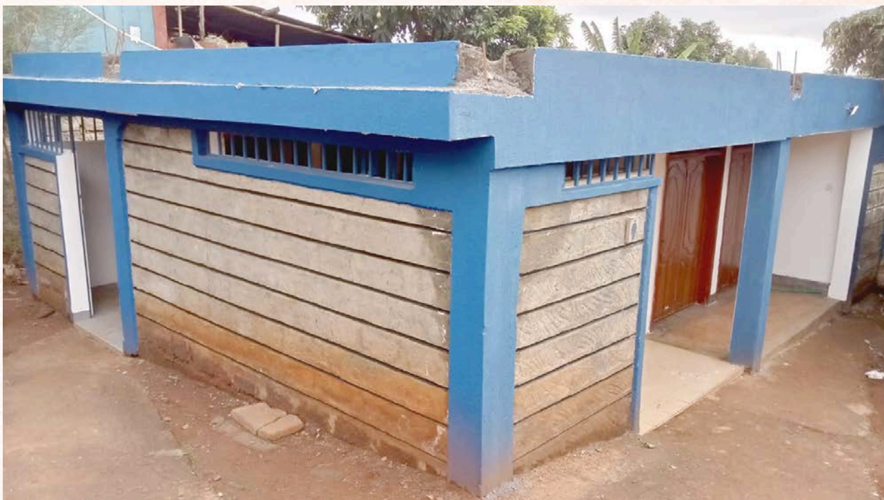
Ablution Block completed
