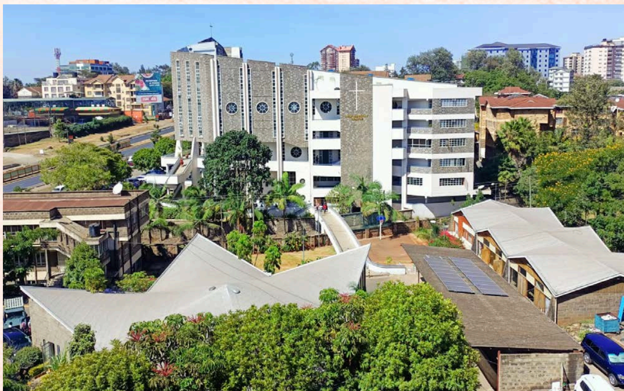
An ariel view of Nairobi Baptist Church
