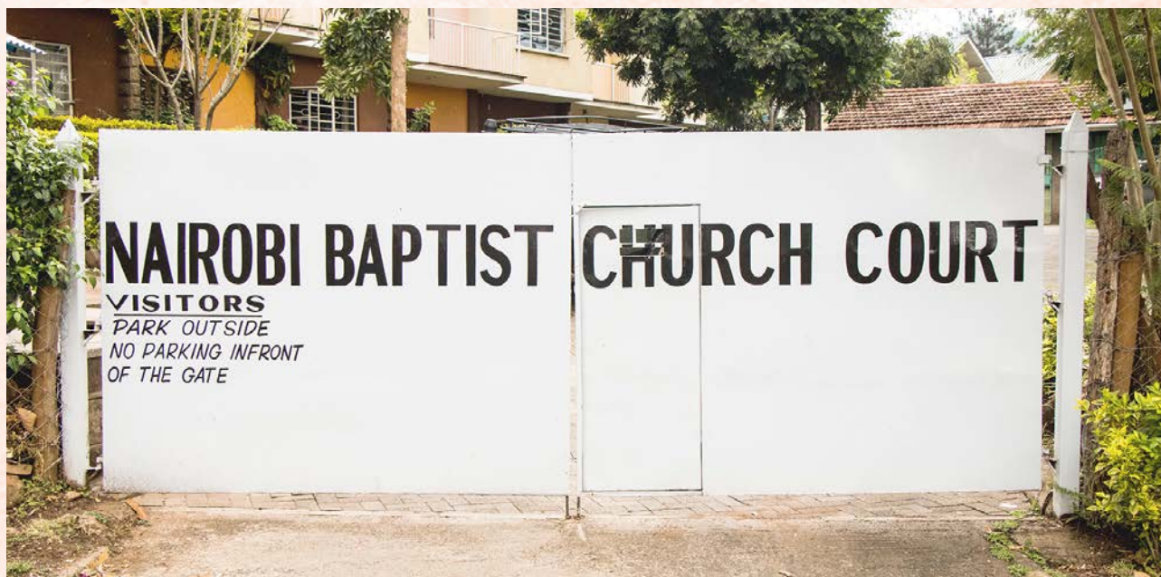
Nbc Court Gate Repaired and Painted
